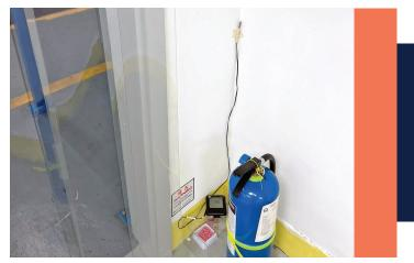
EL-WIFI-TP logger monitoring warehouse temperature
